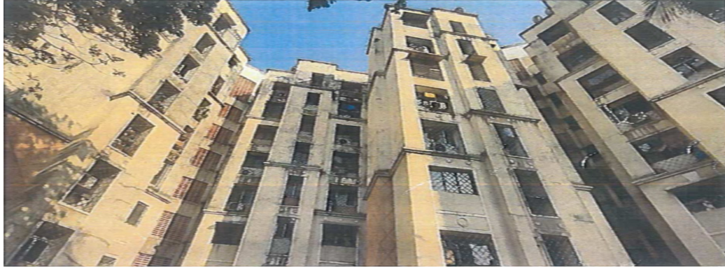
Figure: - 1 Front view of building
